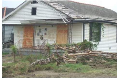
Abandoned house in New Orleans, Aug. 14, 2006
